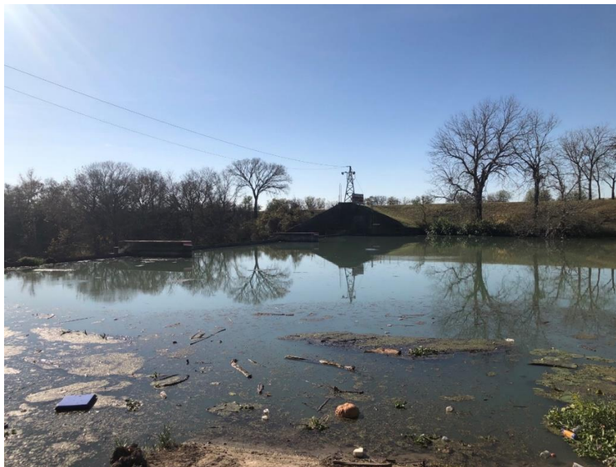
Figure 2-3: Upstream of Nolte Dam (looking downstream from left abutment)
