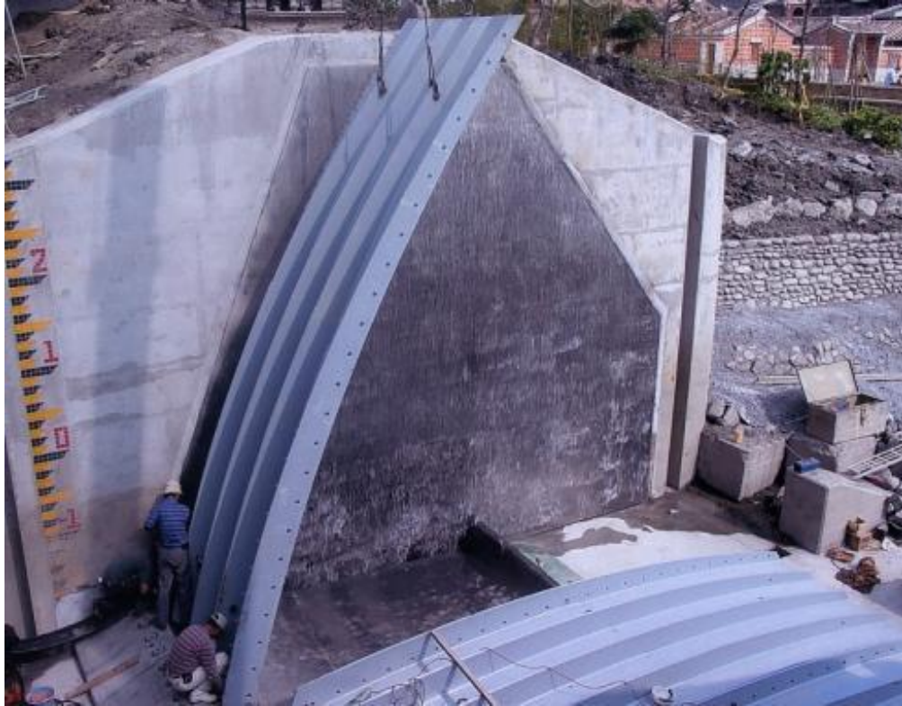
Figure 3-3: Typical Obermeyer Crest Gate Configuration (during installation)
