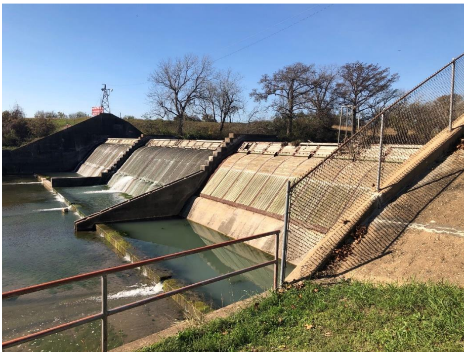
Figure 2-1: Nolte Dam Overview (looking upstream)
