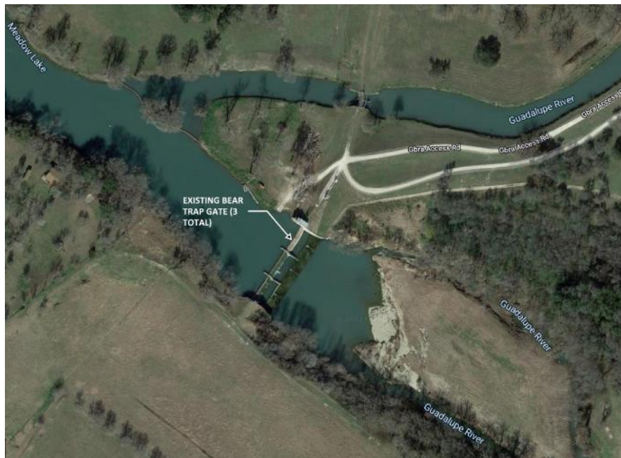
Figure 1-1: Aerial View of Nolte Dam Spillway
